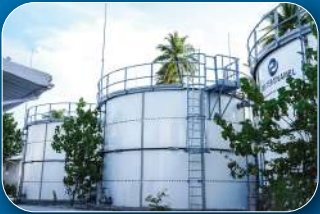
WATER STORAGE TANKS
